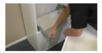
You can then adjust the alignment of the drawers using the controls on the undermount clips to move the drawer box up and down or left and right:
