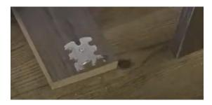
The easiest way to position the bracket is to line it up with the edge of the toe kick and mark the center of your holes 1½" from the bottom of the toe kick:
